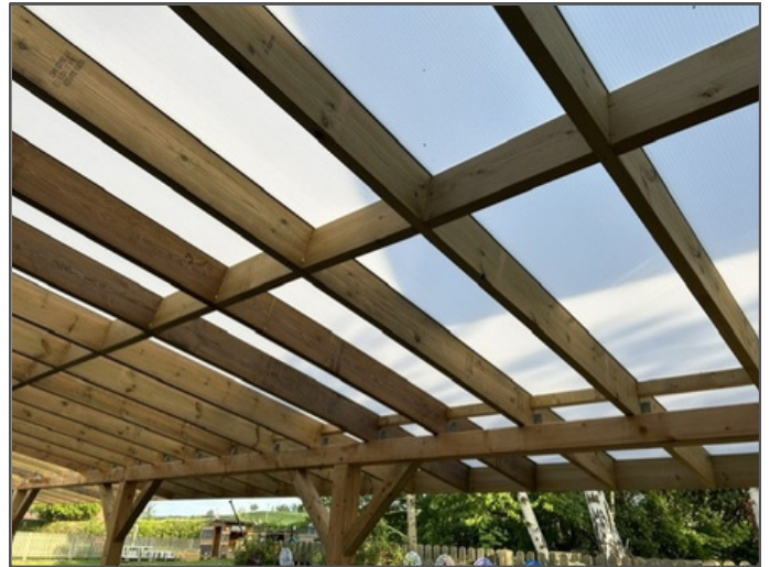
The noggins ensure the timbers don't twist
