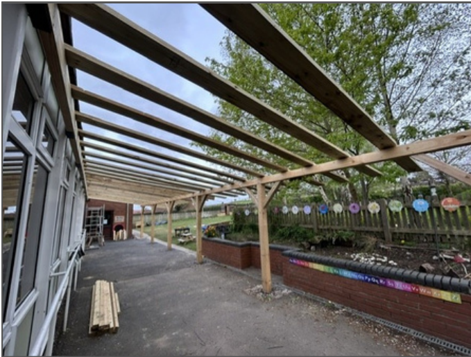
The roof joists go on
