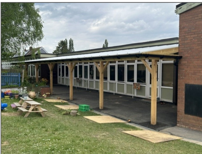
The finished outdoor area complete with UV protected roofing sheets, so it can be used all year round
