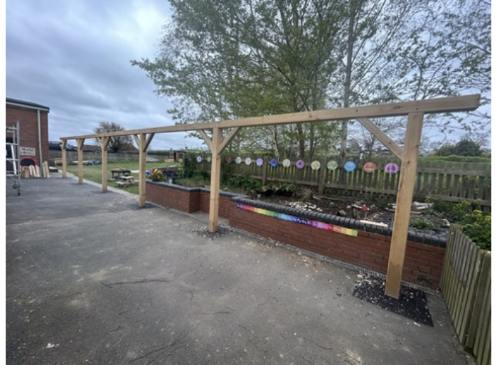
The front timber frame was ready for the roof
